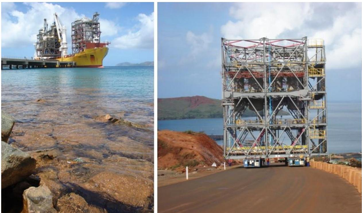
**Figure 2: Modules being offloaded and transportation of module to site**
